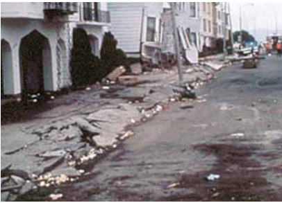
Liquefaction during an earthquake can cause damage of life and property in urban areas as was the case in the Marina District of San Francisco during the Loma Prieta quake of 1989.
